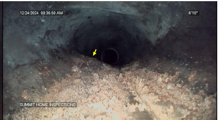
blistered/warped Orangeburg sewer in backyard
