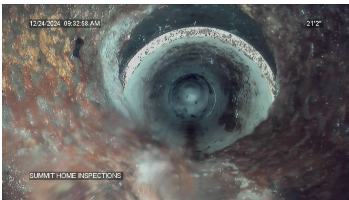
transitions into PVC pipe for city tap; offset noted
