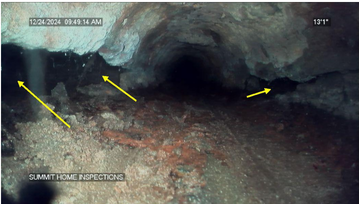
cast iron rotted out on sides of pipe
