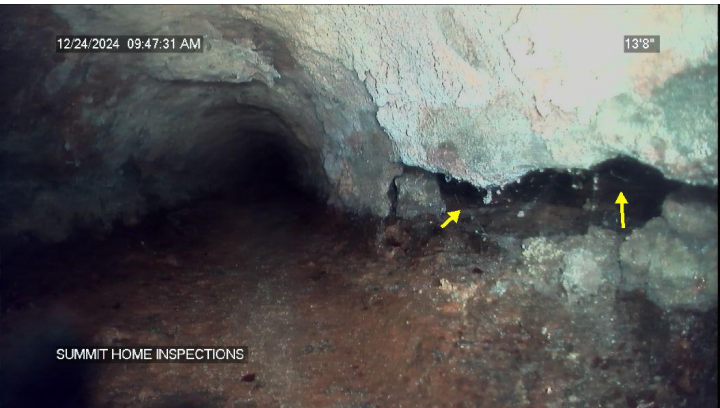
cast iron building drain (under house/slab) with severe rot/deterioration
