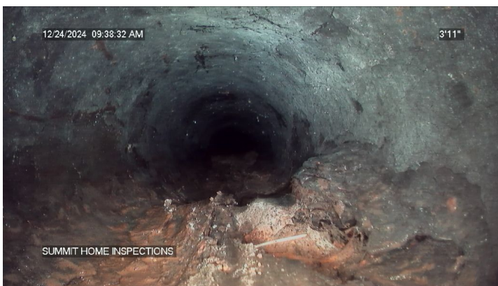
blistering/deteriorated Orangeburg sewer
