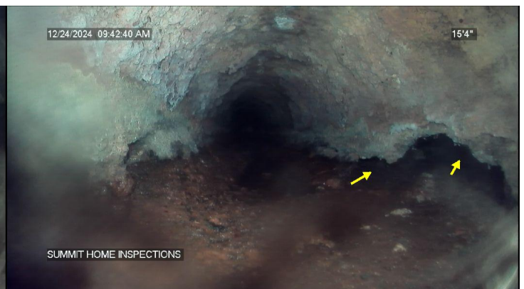
cast iron building drain (under house/slab) with severe rot/deterioration
