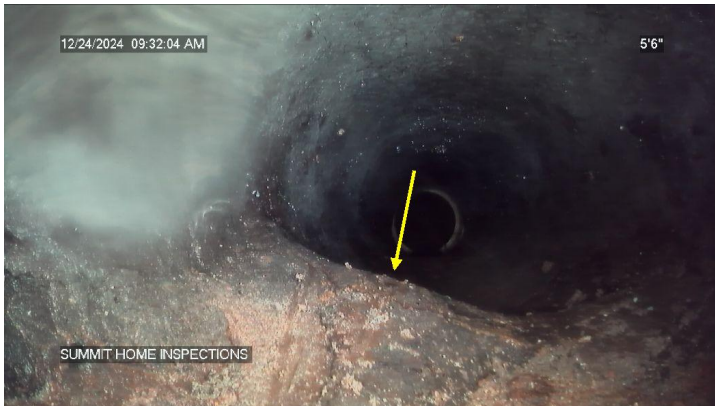
blistered/warped Orangeburg sewer in backyard
