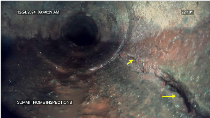
cracked cast iron under house
