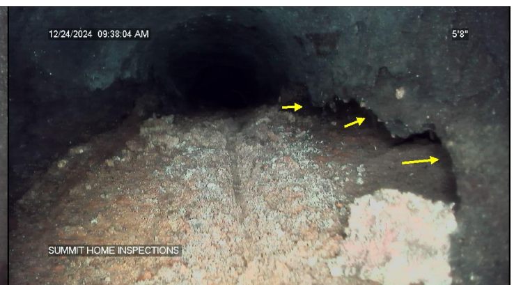
deterioration at sidewall of Orangeburg sewer
