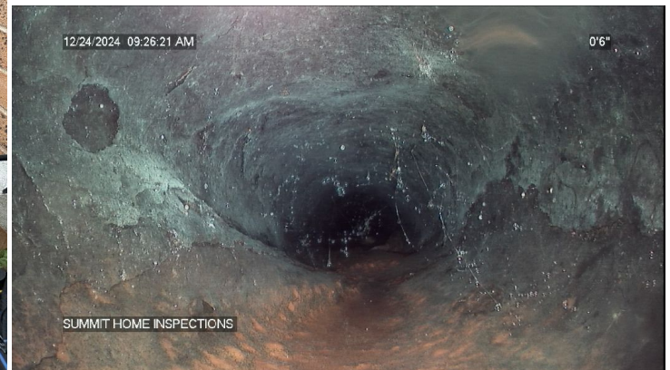
egging/deformed Orangeburg sewer line thru backyard
